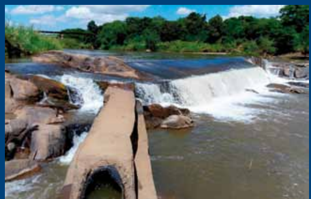
Figure 10.16 Bua River Irrigation Dam in May 2019. © Titus B. Phiri
